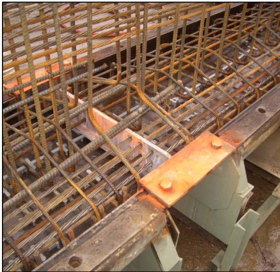
Figure 14: Strand Hold-Up Device
