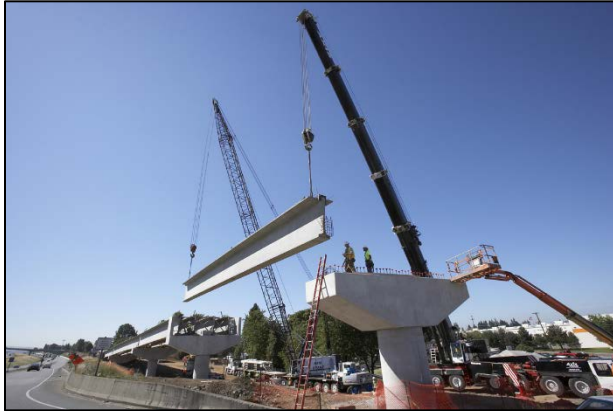
Figure 22: Girder Erection on the Johnson Creek Blvd Bridge
