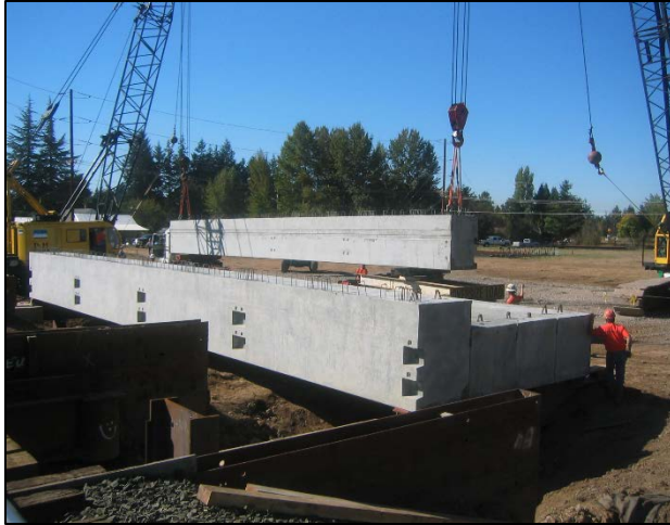
Figure 2: Box Beam Erection
