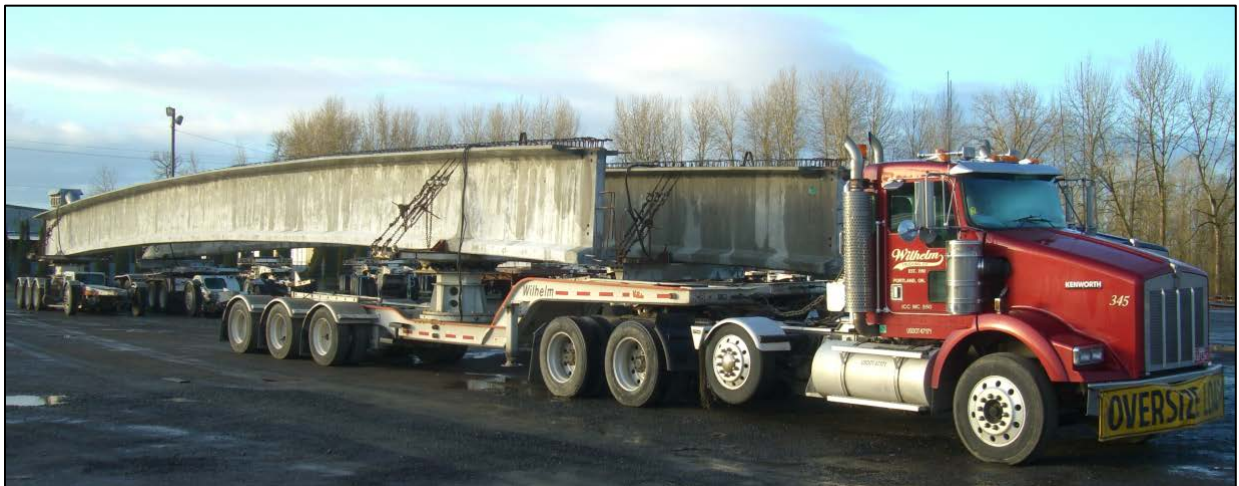
Figure 17: Girders Bunked on Trailers Ready for Shipping
