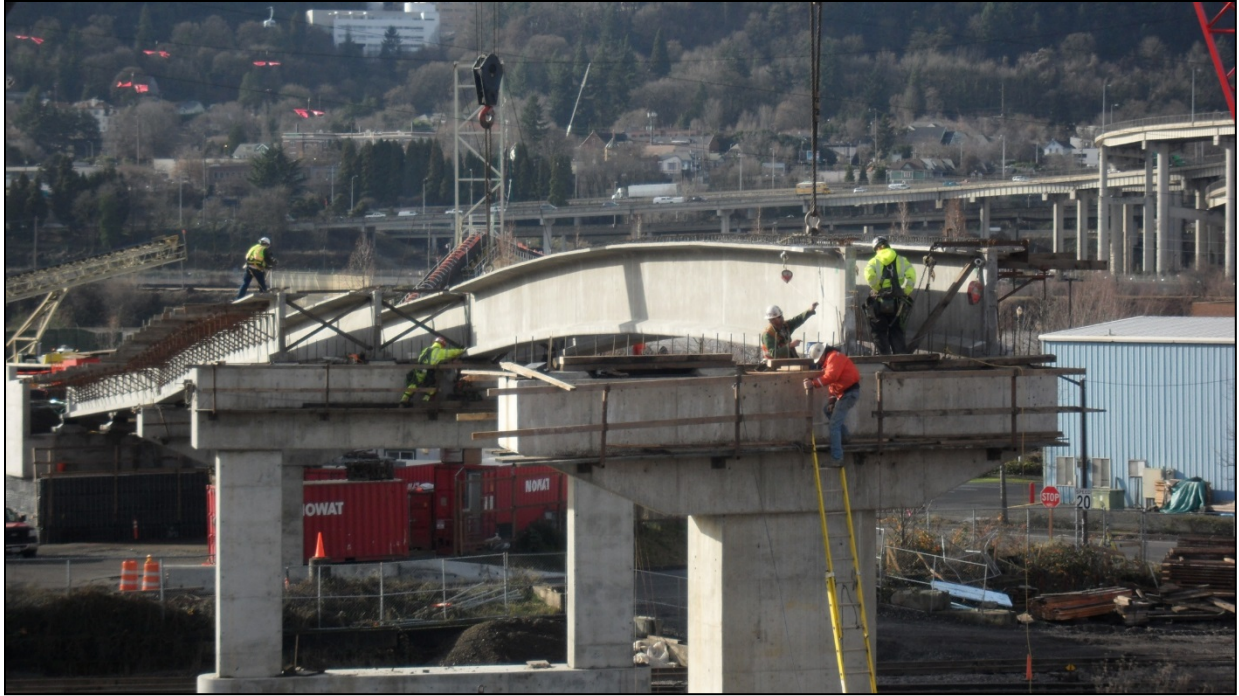
Figure 18: Girder Being Erected Onsite
