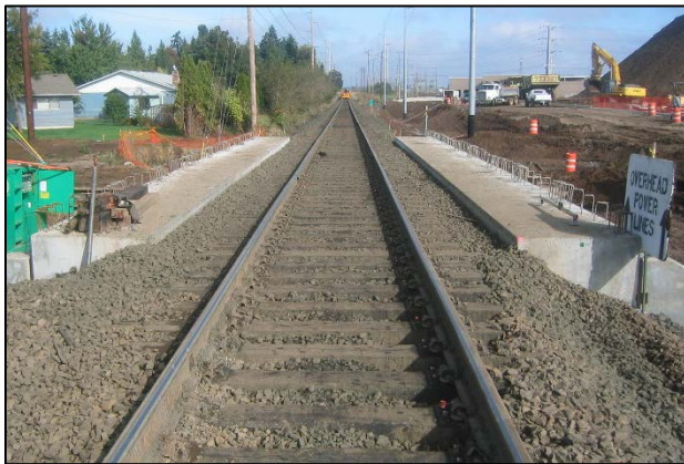
Figure 4: Operational Bridge after Change-Out
