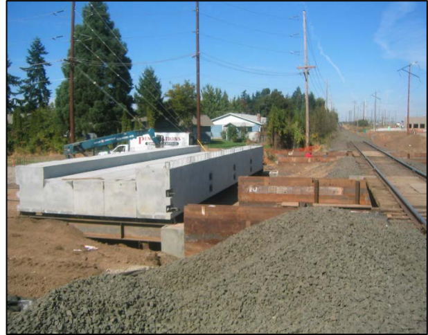
Figure 3: Superstructure Assembled & Waiting to be Moved
