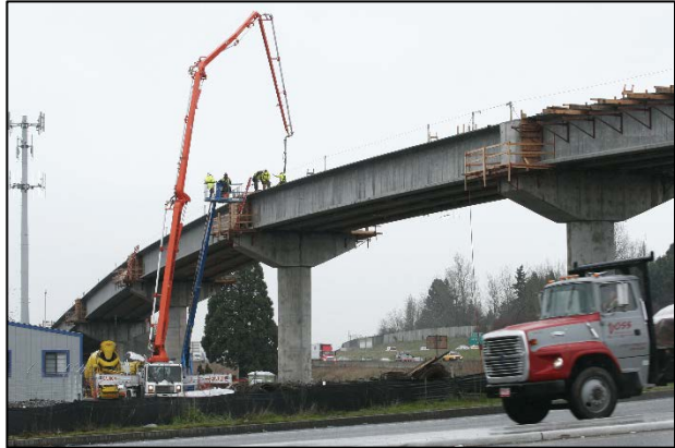
Figure 23: Deck Pour on the Johnson Creek Blvd Bridge
