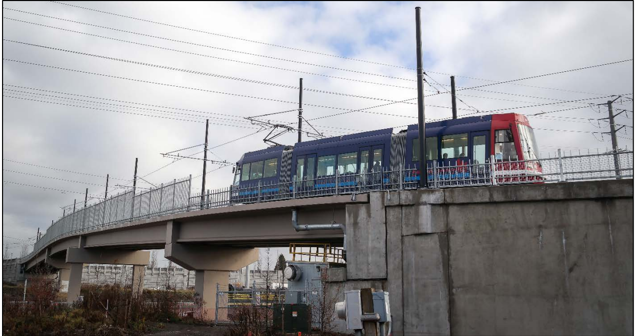
Figure 20: The Portland Streetcar Crosses the Completed Bridge (2)
