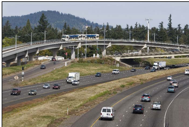
Figure 24: The Completed Johnson Creek Blvd Bridge
