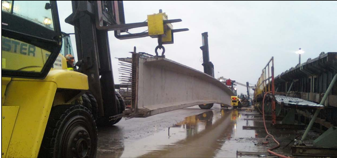
Figure 16: Girder Just After Release of Prestressing Force
