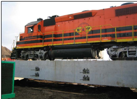
Figure 5: Train Crossing Bridge Prior to Excavation
