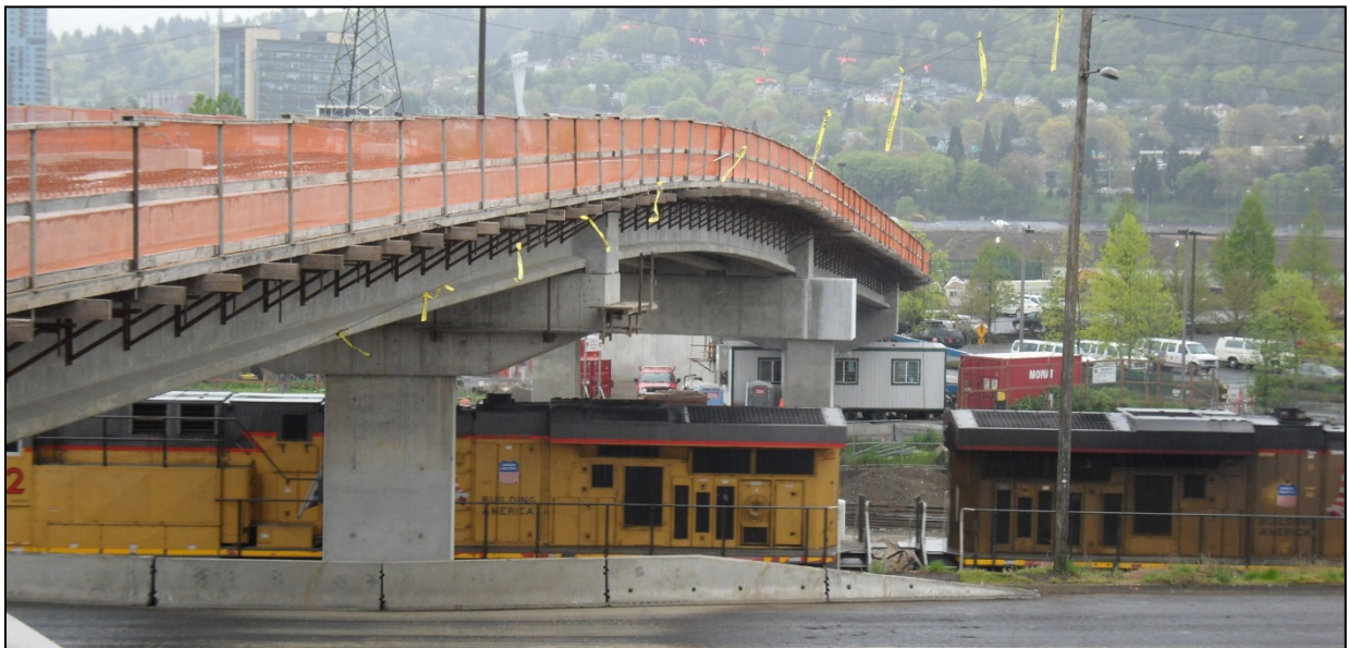
Figure 19: UPRR Train Passing Underneath Span 2
