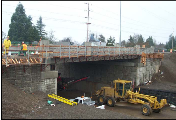
Figure 6: Roadway Construction Underneath Bridge
